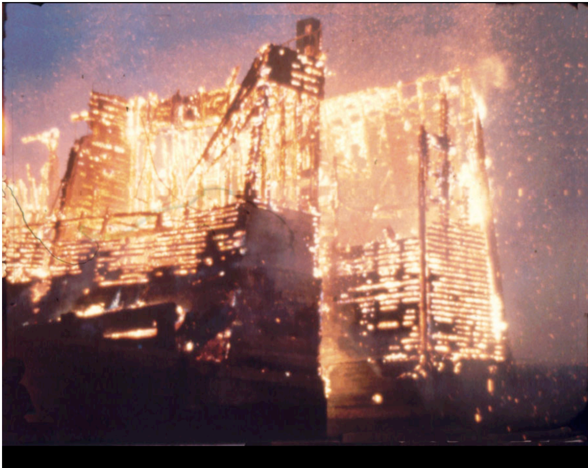
The 8 inch thick walls evaporate
